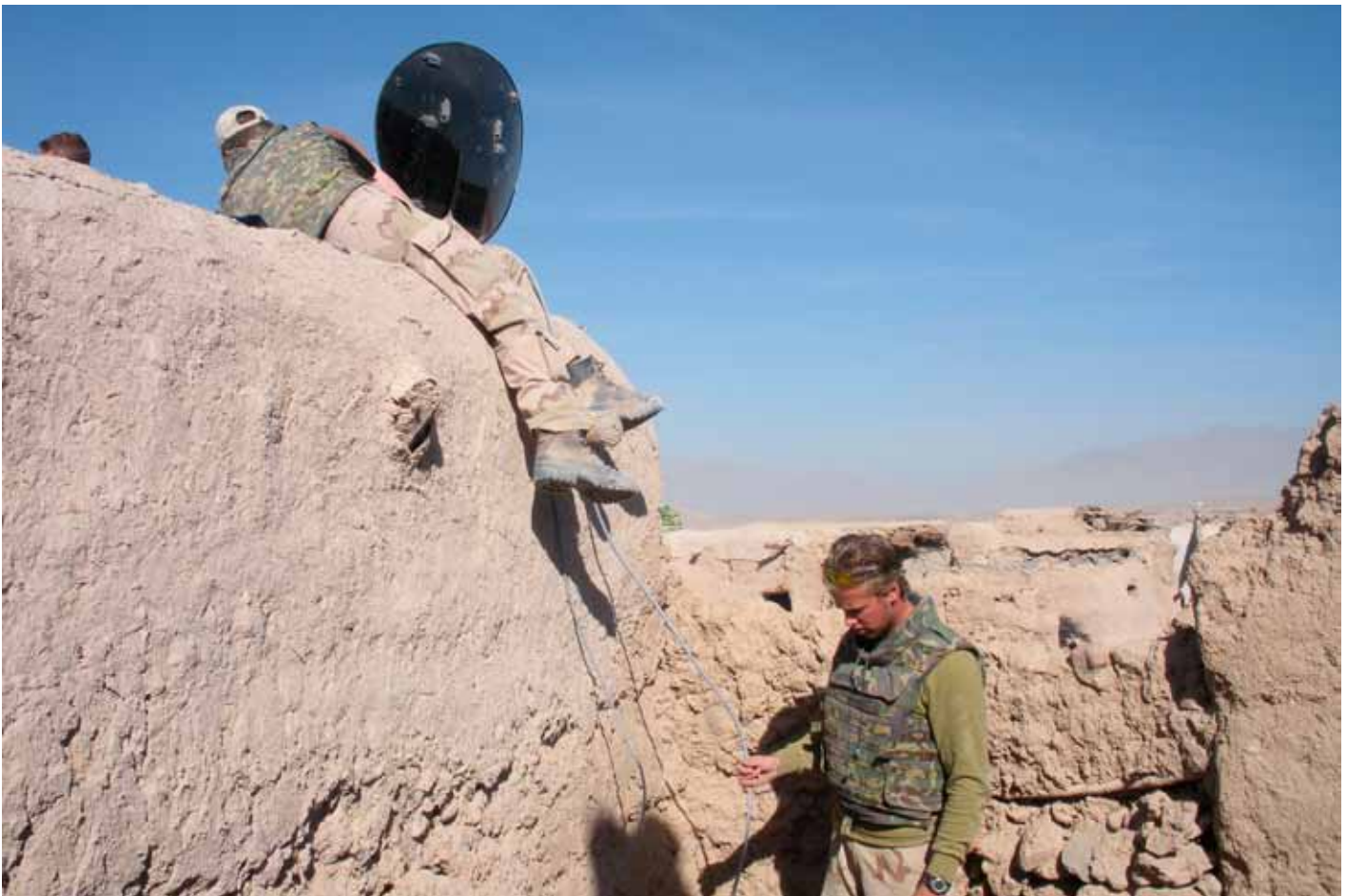
Installing Tactical Comms on Forward Operating Base
