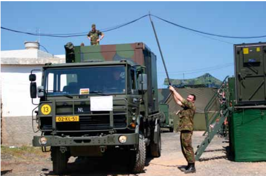
Tailormade cabling and installation
