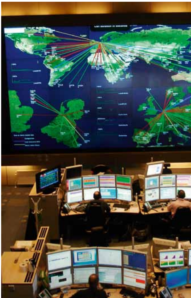
KPN Network Operations Center
